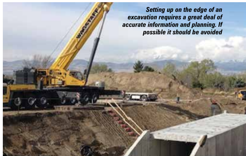
The ground in this marina was not as compacted as reported. This coupled with a deviation to the route caused the retaining wall piles to give way and the crane to end up in the water
