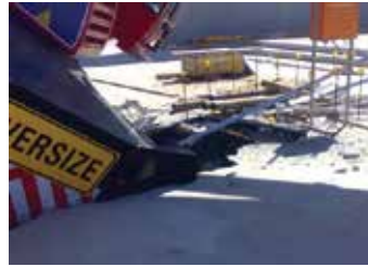
This 250 tonne crane found the one missing deck support prop among hundreds.
