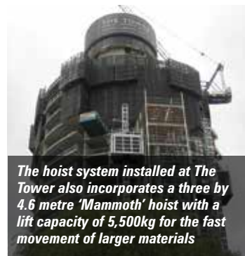
The 100 metres per minute, 3,200kg capacity Scando 650 FC-S 100 - are specifically designed to speed up construction time and save costs with a full height transit time reduced to just 90 seconds
