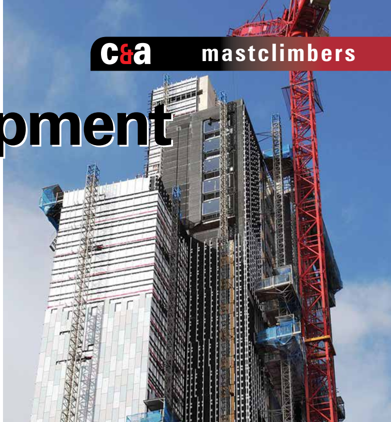
Of the 17 platforms six were 'double deck' - two independent platforms on the same mast - allowing two different operations to take place simultaneously.
