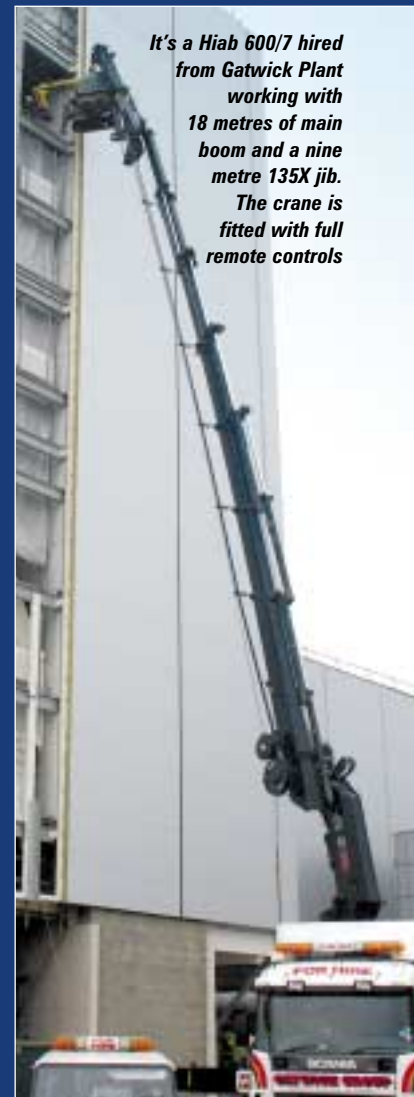
A special self propelled cutting tool is lifted into an upper floor for refit work at a Gatwick airport pier. What crane is it?
