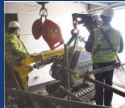
A special self propelled cutting tool is lifted into an upper floor for refit work at a Gatwick airport pier. What crane is it?
