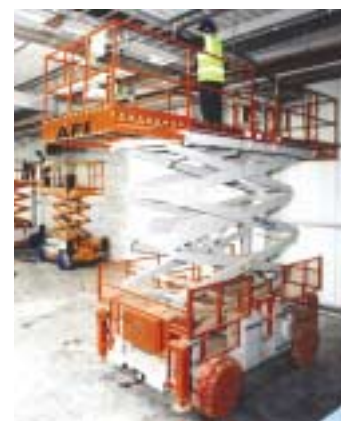
If you are using larger scissor lifts with black tyres and are concerned about your floor, insist that they are fitted with socks like these units, working on electrical installation at a new car parts manufacturing plant in Derbyshire.
