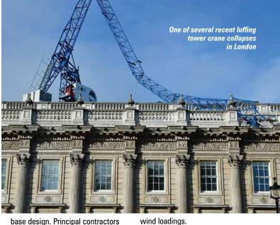
base design. Principal contractors have primary responsibility on site, and they must liaise with subcontractors, crane owners and crane operators to ensure that when left unattended in the out-of-service condition, all tower cranes must be configured correctly to withstand
