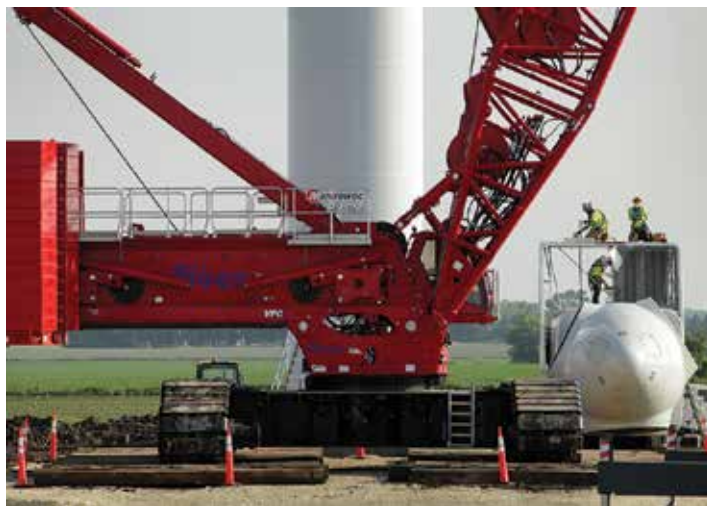
The VPC system automatically positions the MLC650's counterweight to suit each lift.
