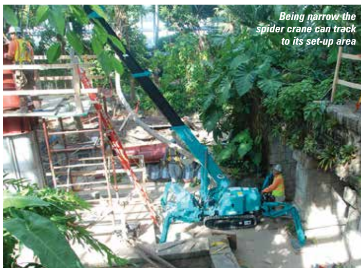
A Reedyk C3412 Compactcrane working in a very tight space
