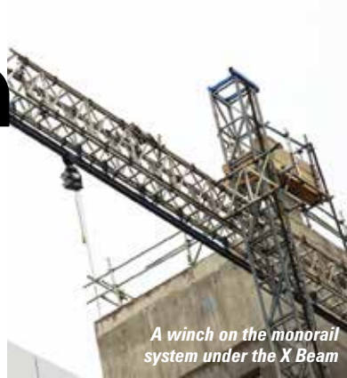
The innovative use of mastclimbers to span across a main road gave access to both sides of the viaduct for strengthening and repair works. This access solution saved the customer eight weeks on his program and 40 percent of the budget had a conventional scaffold been used
