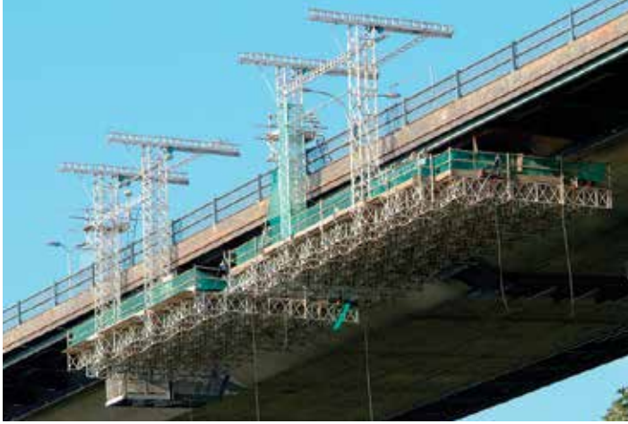
Four platforms were installed on the Erskine Bridge over the river Clyde in Scotland (two at each side). The leading platforms on each side allowed the removal of the old runway beams with the materials handling system while the two following platforms provided access for fitting new runway beams.
