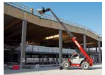
A-Plant has spent £3 million on Manitou telehandlers.
