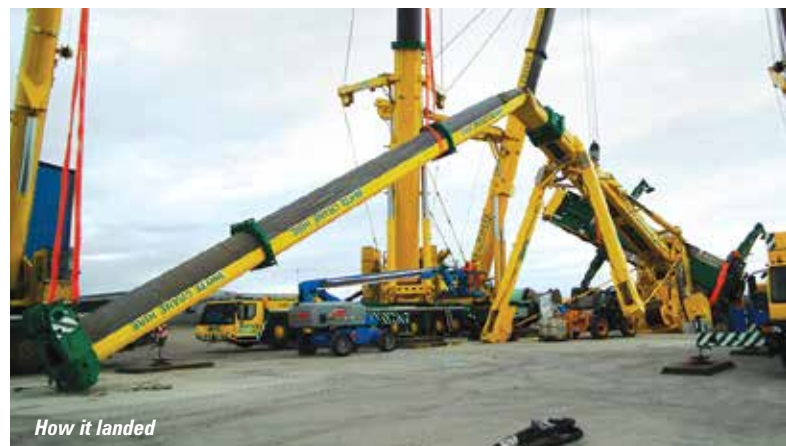
The crane is finally lifted and rotated
