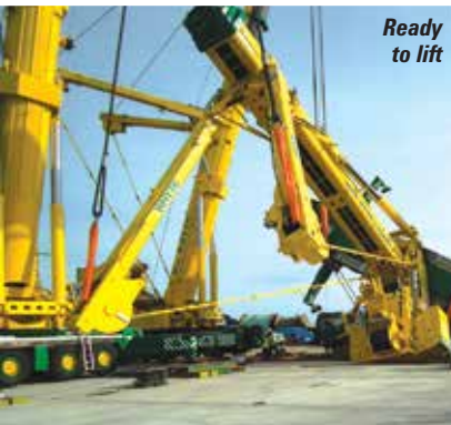
One of the four collars - each weighing two tonnes
