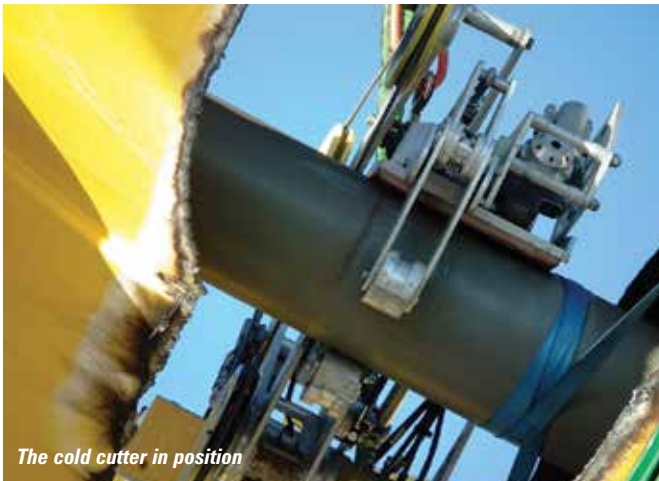
The cold cutter with the telehandler drip tray underneath
