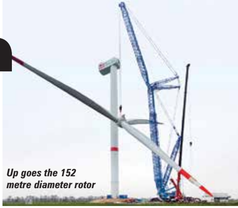
Three crawler cranes were used to place more than 2,600 pre-cast concrete components
