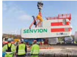
The massive turbine housing weighed 220 tonnes with hook and beam.
