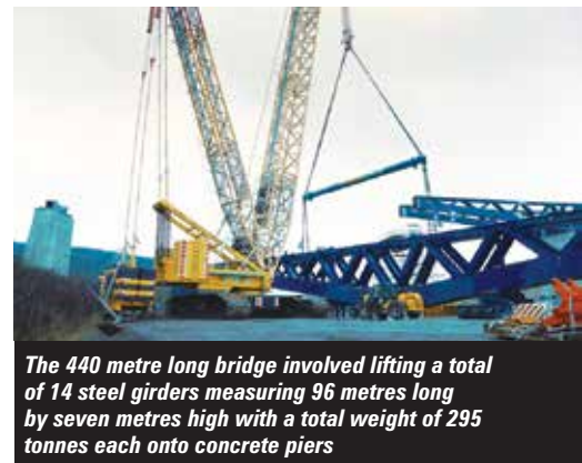
Using the LTR 1220 as counterweight significantly reduces the amount of ballast required on site
