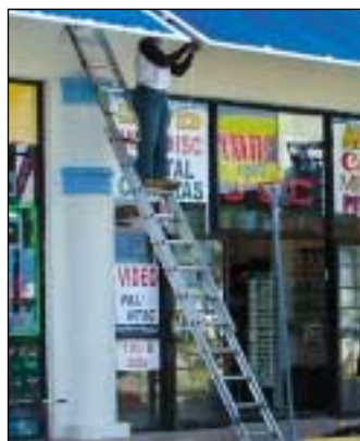
How not to use a ladder! A large number of serious injuries and even fatalities occur below 3m.
