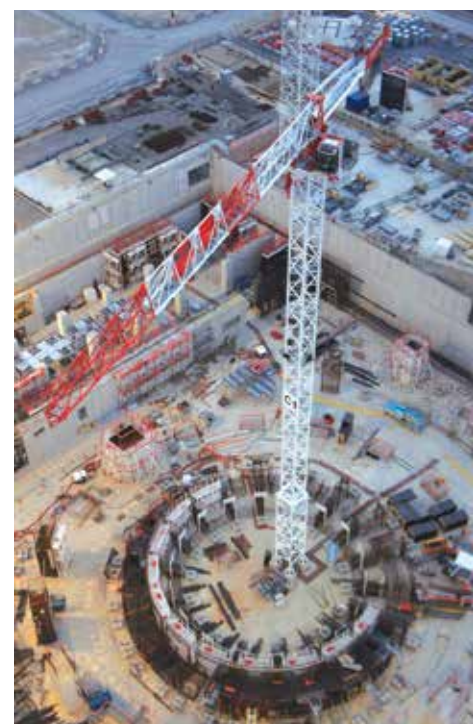
Six Potain cranes - two topless and four traditional top slewers - are helping construct the €300 million ITER fusion reactor in the South of France.
