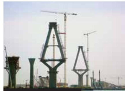
The two main bridge pylons are 185 metres high
