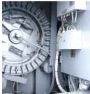
Electrical system is renewed hydraulics revised
