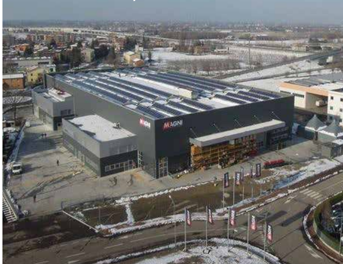
The all new 6,000 square metre facility in Castelfranco Emilia near Modena in northern Italy
