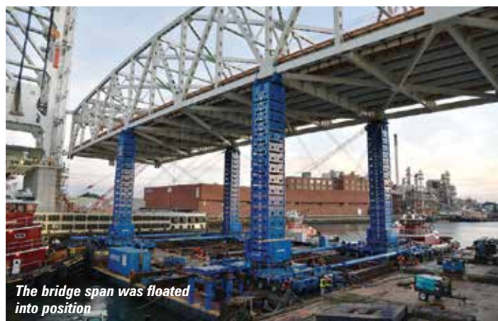
The new lift bridge span almost in position
