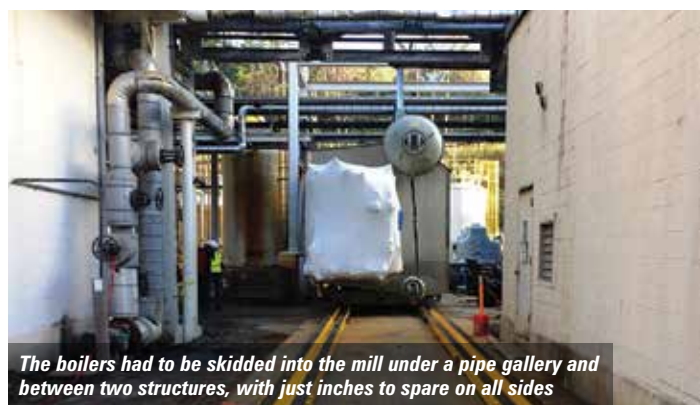
Once the boiler was off the railcar it was lifted by a Grove GMK 7550, slewed through 90 degrees and installed on the skidding system
