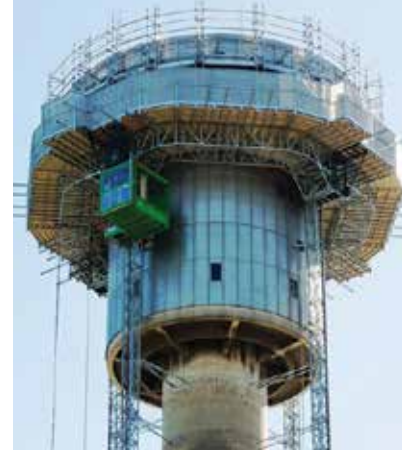
A circular demolition platform in Sydney
