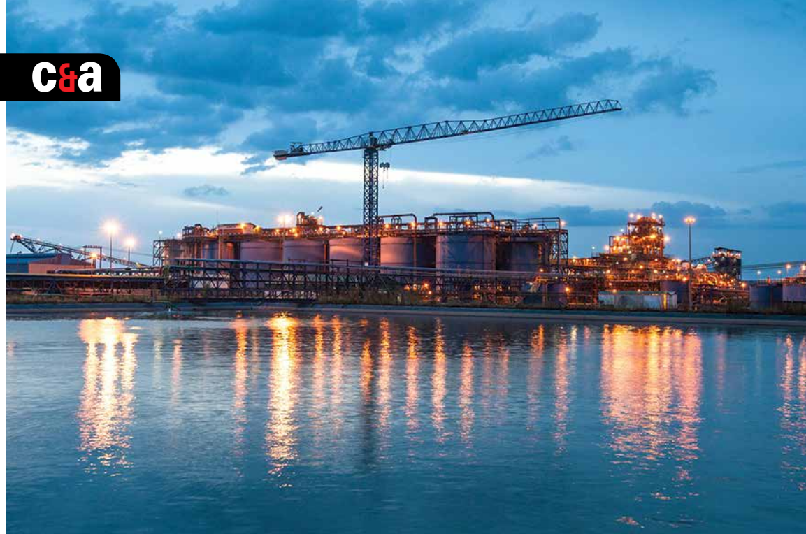
The Hup 40-30 has a 40 metre jib lifting one tonne at the tip
