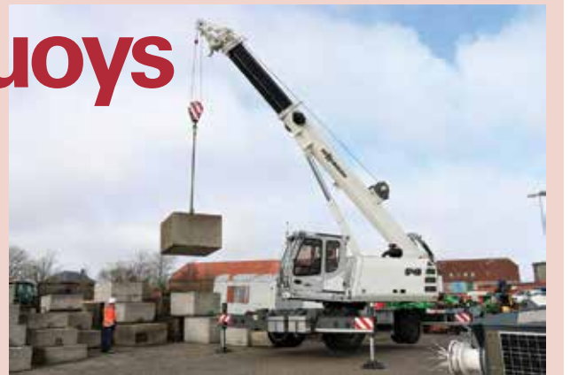
The Sennebogen 643 is used to manoeuvre all buoys at WSA Tönning
