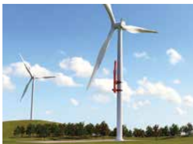
The 100 tonne WTM 100 pulls itself up on pre-installed lift rings and then clamps to the tower before lifting.
