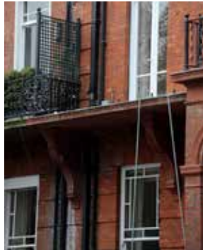
The cast iron balustrade gave way.
