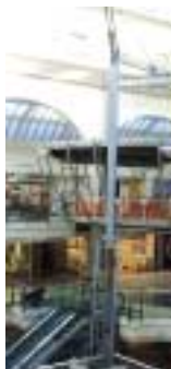
Look down from above and a crane is revealed.
