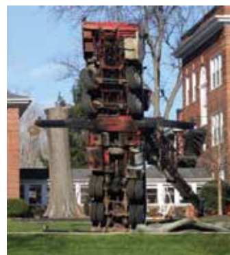
A crane operator should know how to calculate the approximate weight of tree sections - getting it wrong can have serious consequences.
