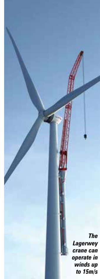
The Lagerwey climbing crane undergoing testing
