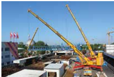
The main girder had to remain suspended in position for several hours.
