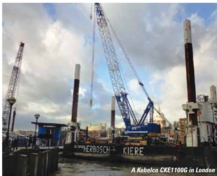
BPH's CKE1350 working on a flat top barge
