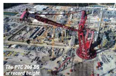
Mammoet executing the wash tower lift
