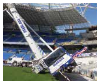
A soft verge takes another crane
