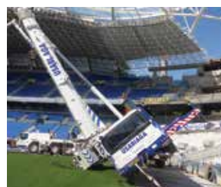
A soft verge takes another crane
