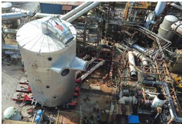
Mammoet designed a jack and slide system that could cradle both the old and new vessels at the foundations to elevate and slide them into place.
