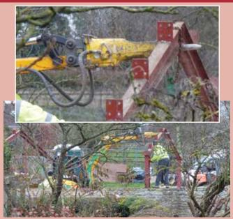
Spotted in the UK a demolition contractor dismantling a steel frame building using an excavator and breaker for all the lifting. As they removed the bolts from the joined roof truss, it rotated on the breaker tool wildly, almost knocking one of the men in the head and brushing the other off the wall he was standing on.
