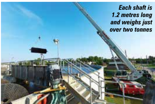
The 75RT was able to fit into the limited space available between the tank wall and the perimeter fence
