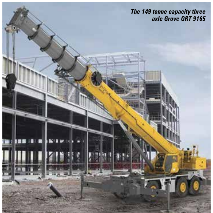
Two 45 tonne Ormig cranes
