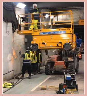
Spotted in a tunnel in what looks like the UK, a team working at height with a scissor lift and telehandler. For some reason they have lifted a stowed 26ft scissor lift with a compact telehandler to reach a light at a height of around five metres. It looks as though none of the crew question the methodology.
