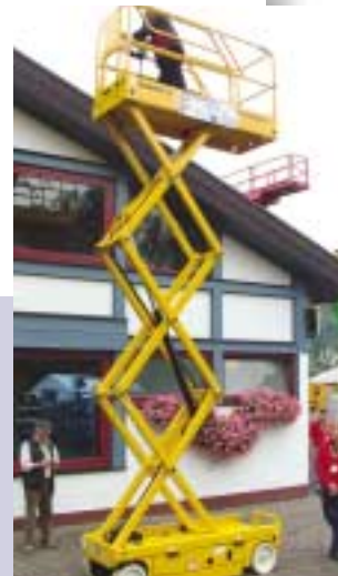
The Haulotte platform height is checked.
