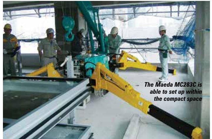
The curtain walling panel almost in place
