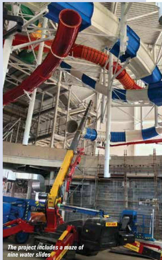
Work was carried out at various levels within the water park
