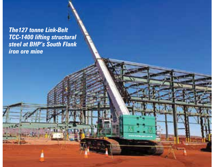
The TCC-1400 has a 59.5m main boom with a 78.5m tip height
