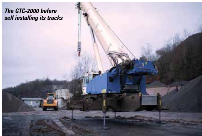
The GTC-2000 has 50 percent gradeability, 420mm ground clearance and weighs just under 150 tonnes
