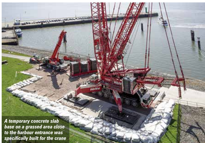
An eight axle 750 tonne Liebherr LG 1750 truck crane was chosen for the lifts
