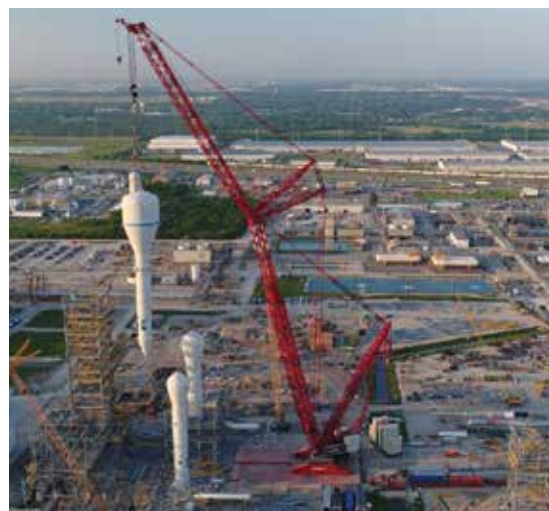
Mammoet used just one heavy lift crane - a 3,200 tonne Liebherr LR13000 - at Braskem's new $675 million Gulf Coast polypropylene plant at its Delta facility in La Porte, Texas.
