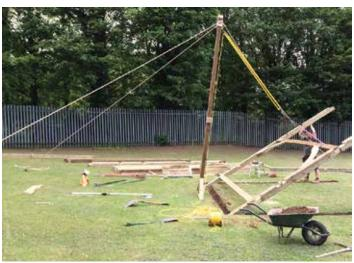
corresponding pole angle. Correctly rigged these adjustments may be undertaken while under load by the simple use of pulleys or hitches in the guy line system.
