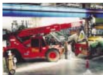
A typical shifting job
