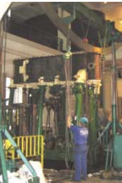
There was Barely an inch of headroom for this lift.
