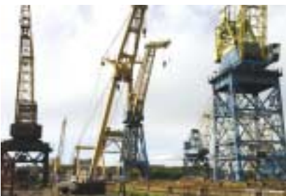
Taklift 4 takes the strain at Wallsend
