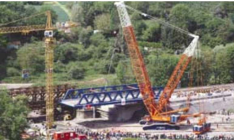
The Liebherr LR750 travels off centre with its 325 tonne load avoiding a tower crane.
