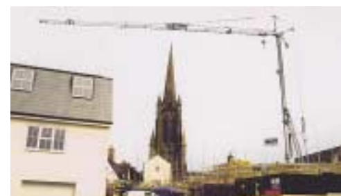
The Vanson VC30 was chosen for this siter in Bury St Edmunds thanks to its smooth start controls.
