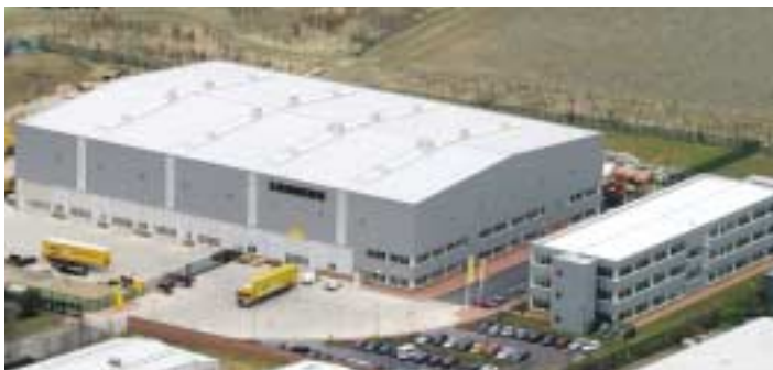
Liebherr GB's new Biggleswade facility
