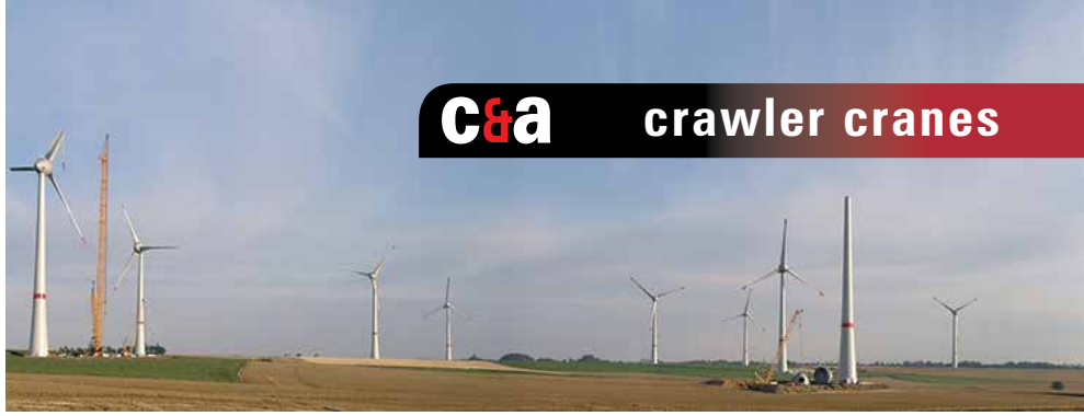
Telescopic crawler cranes, such as this 220t Liebherr LTR 1220 are ideal assist cranes on wind projects
