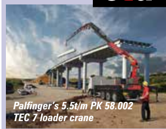
Palfinger's 5.5t/m PK 58.002 TEC 7 loader crane
