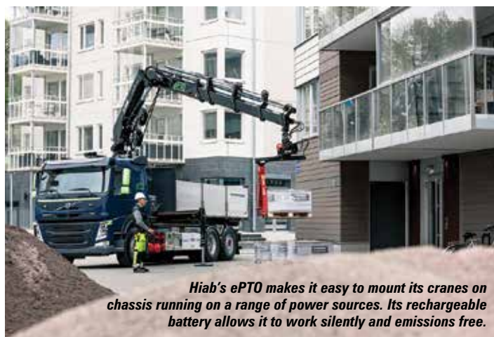
Kynningsrud puts the first Liebherr Unplugged crane to work
