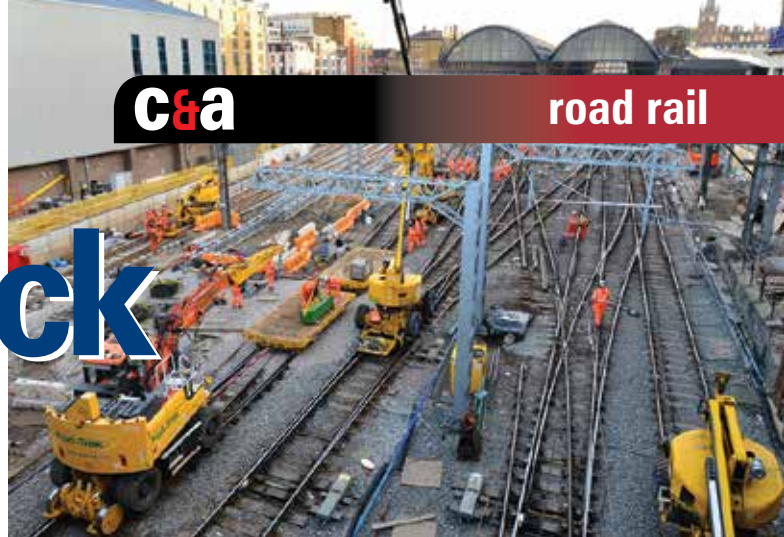
Suppliers of rail mounted equipment must often work at night while lines are closed. TXM's 'Monster Crane' can pick & carry loads from the nearest road access point
