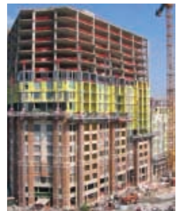
Scaffolding for a 10- to 12-storey block on four sides can take up to four to five weeks to erect and up to four weeks to dismantle. To cover the same building with MCWPs would take about a week.
