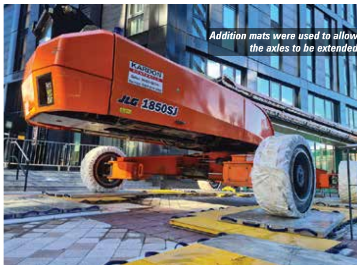
The JLG 1850SJ moves into position
