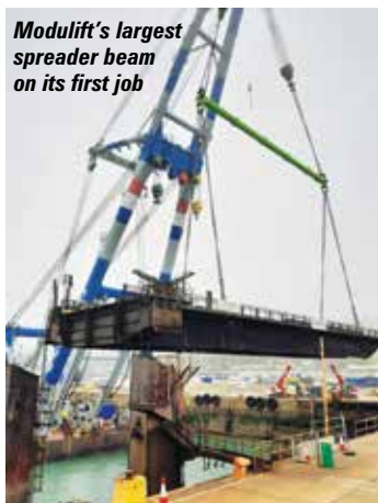
The 2,000t MOD 1100/2000 combined with two 400t Modulift MOD 400 spreader beams
