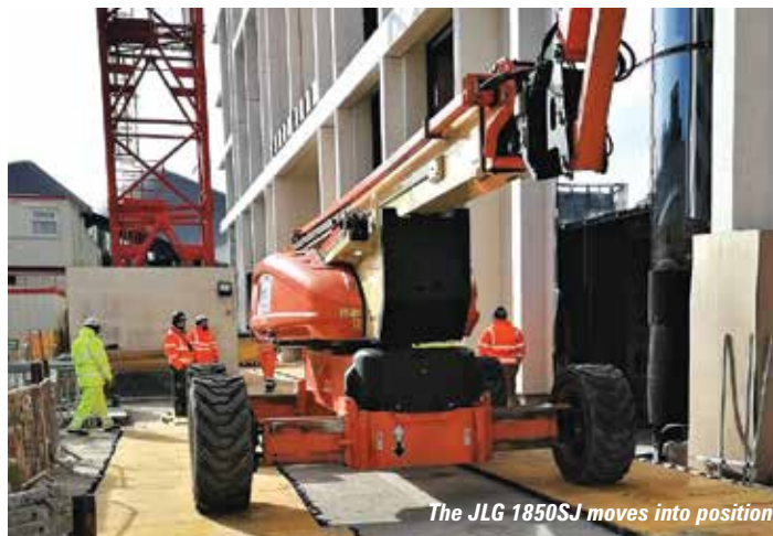
Addition mats were used to allow the axles to be extended
