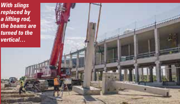
...and installed in the ground
