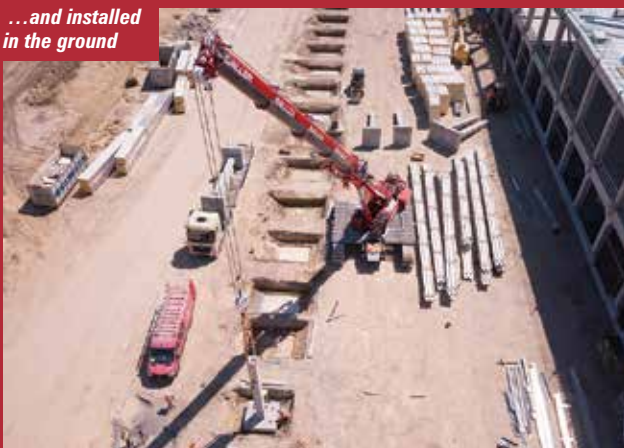
Saller installed 210 columns and 2,400 concrete components for the warehouse
