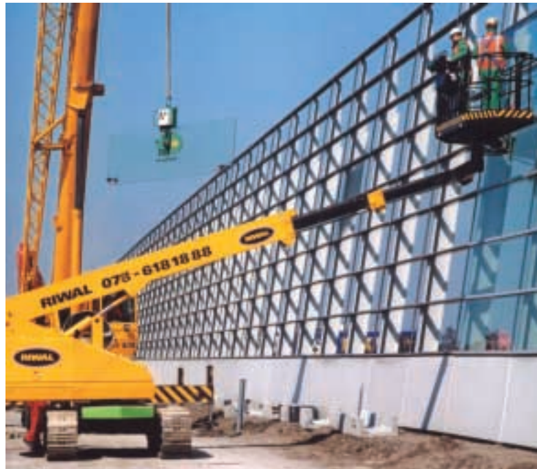
Aichi booms are being used on Holland's motorways to install sound suppression a number of the units have special 4x1m platforms.
