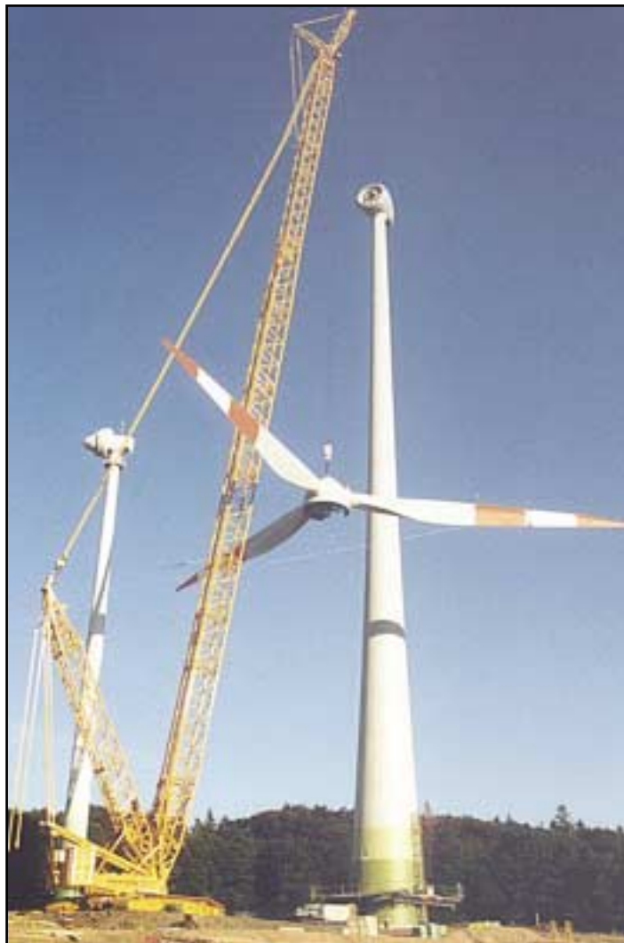
A typical example of a two-line lift is that of a windmill's rotor blade.
